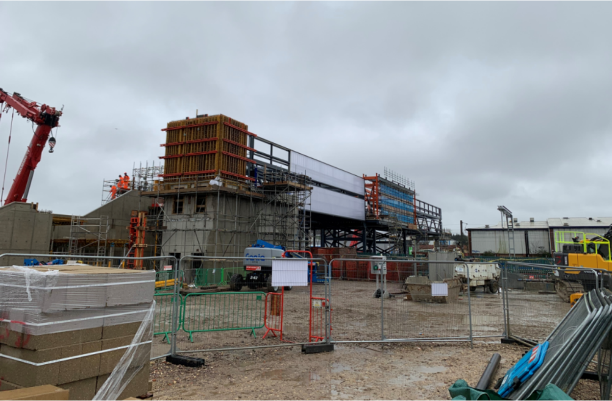
Eastern entrance lift shaft and footbridge partially clad
