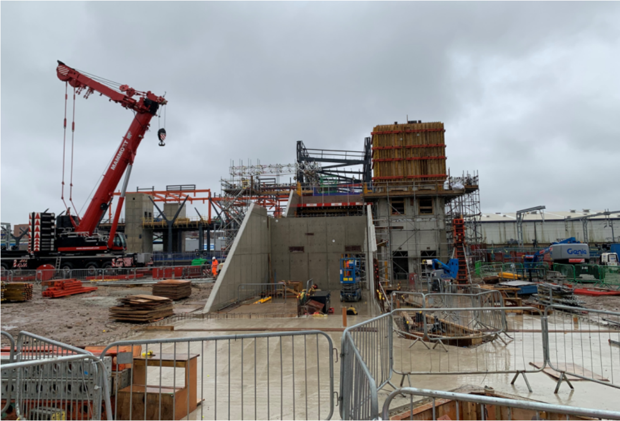
View of Eastern entrance looking east to west
