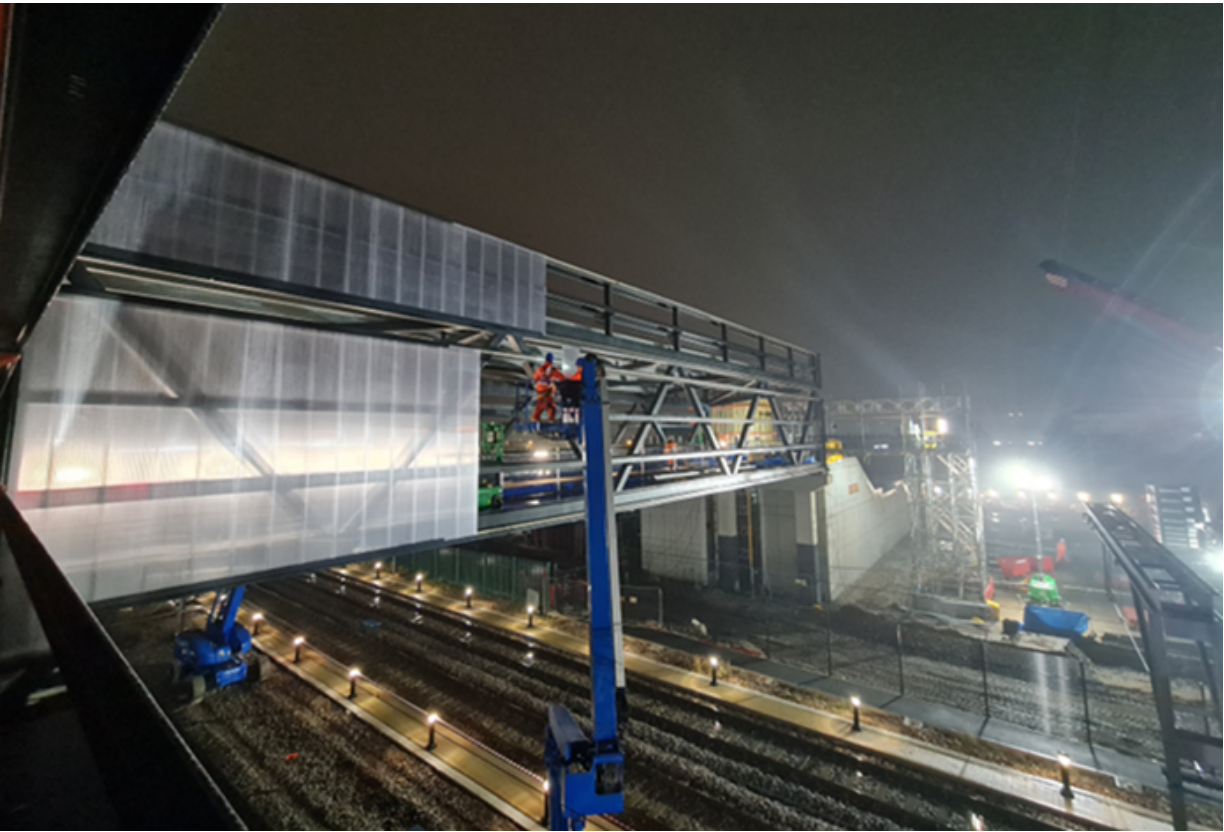
Footbridge cladding underway
