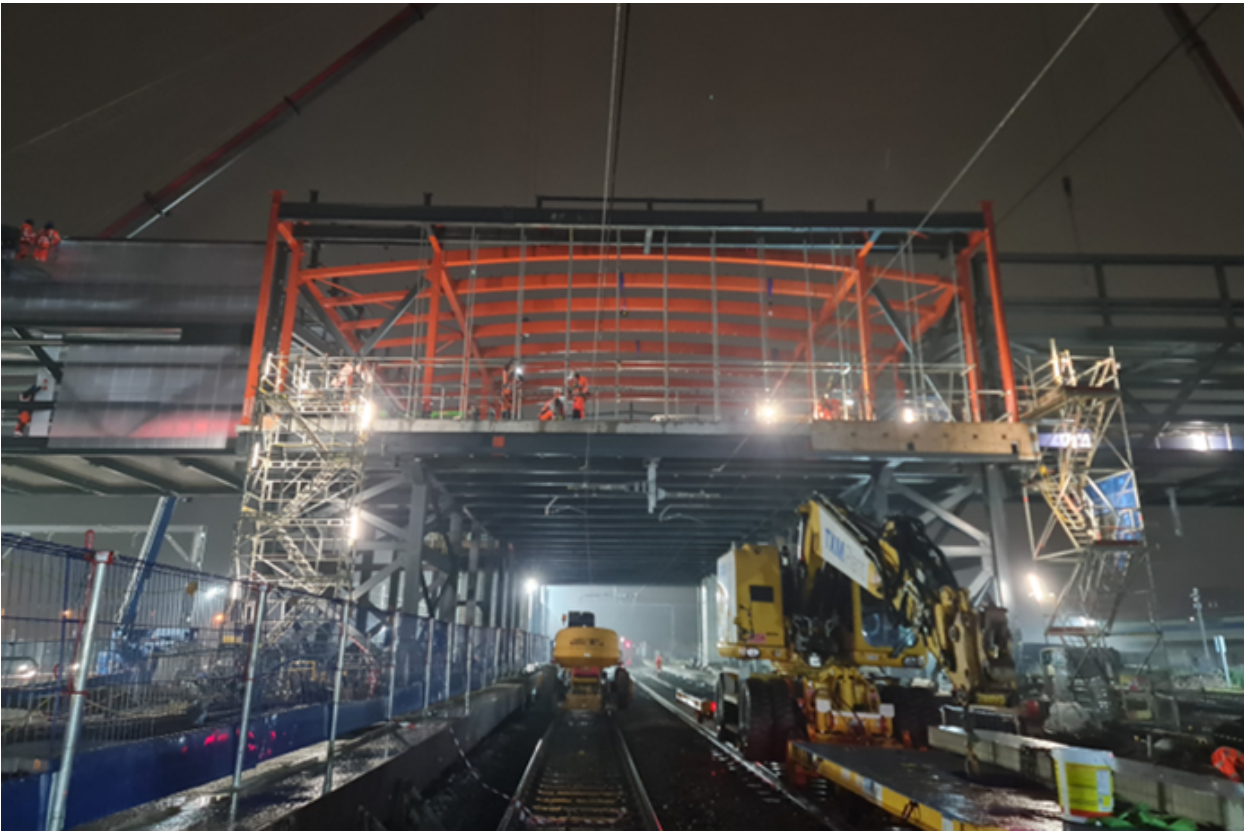
View of station concourse from below
